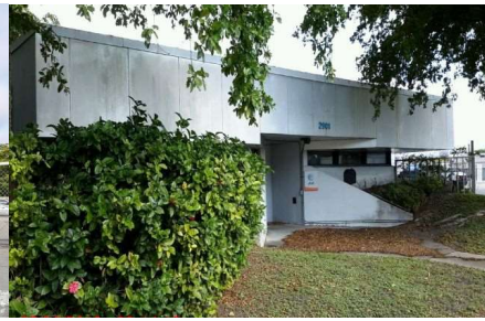
North West View
